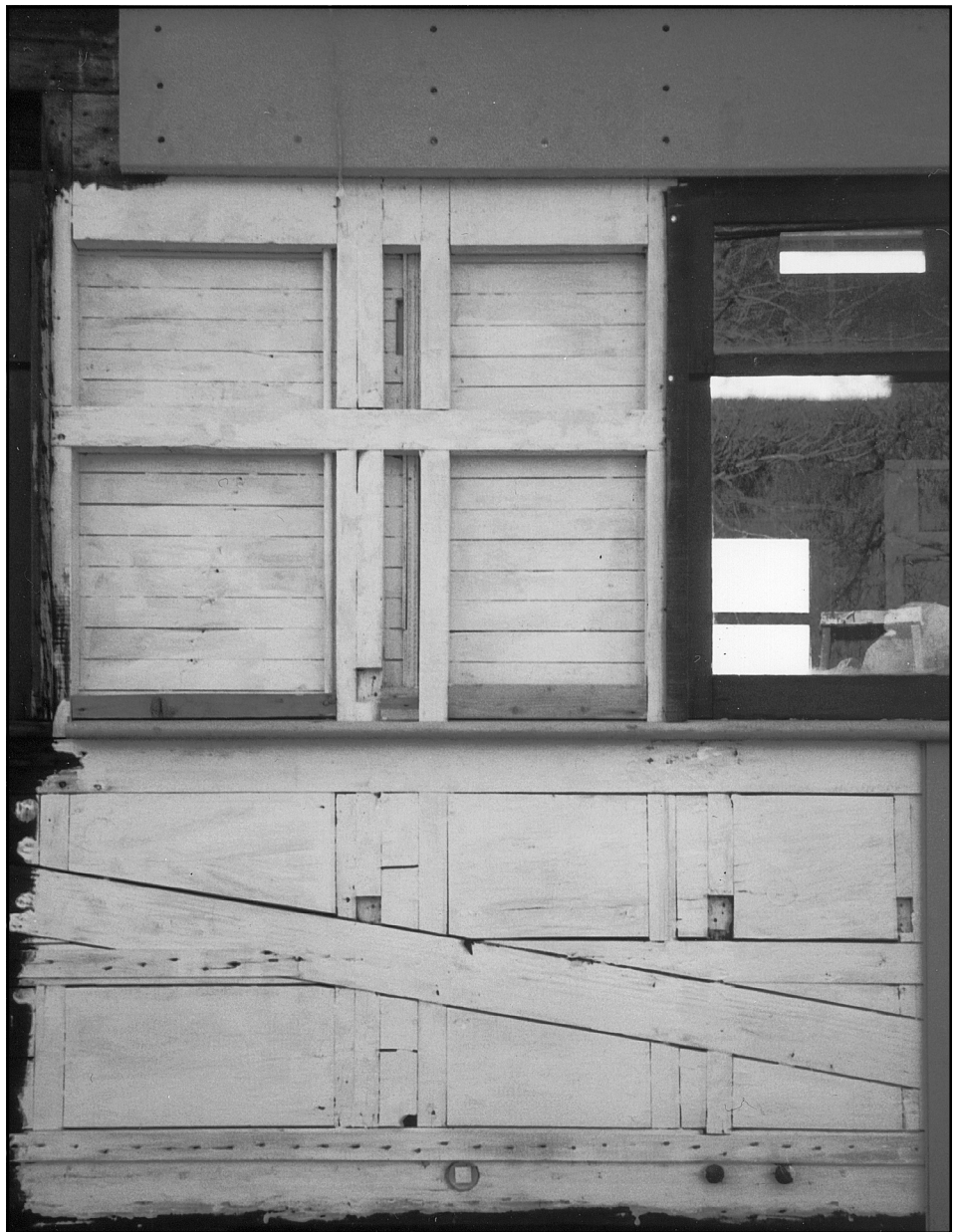
The Rico's side framing is exposed during siding replacement. You can see that the area below the window is completely filled with wood. The new fascia board and window frame are also in place. – Two photos © Bob Tully.
