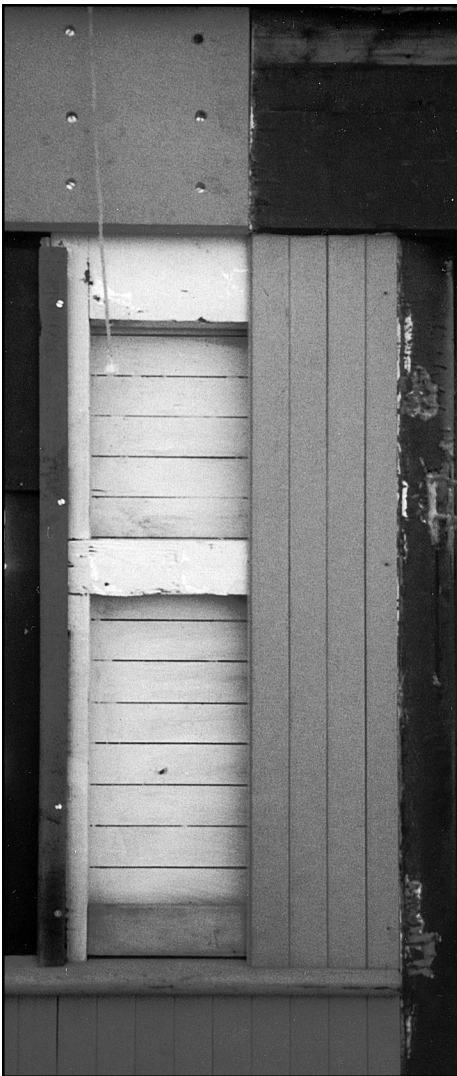
A new fascia above, new siding, new window frame and a new sill improve the north side of the Rico.
